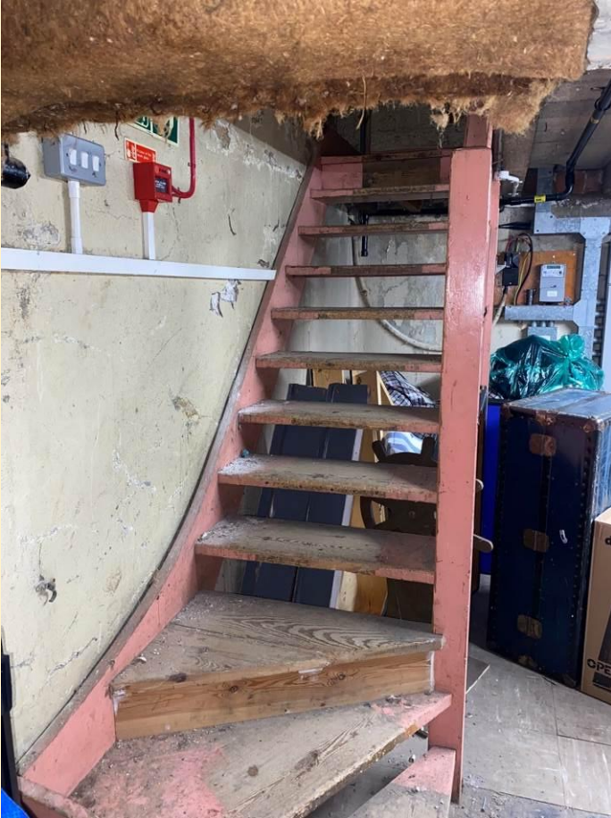
Narrow staircase to Basement
