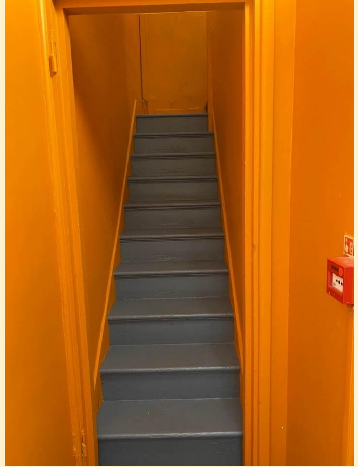
Narrow staircase to First floor
